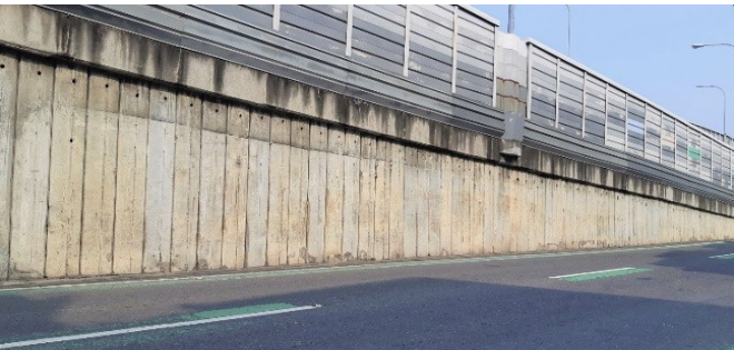
Fig. 2-5 Roadside retaining wall
