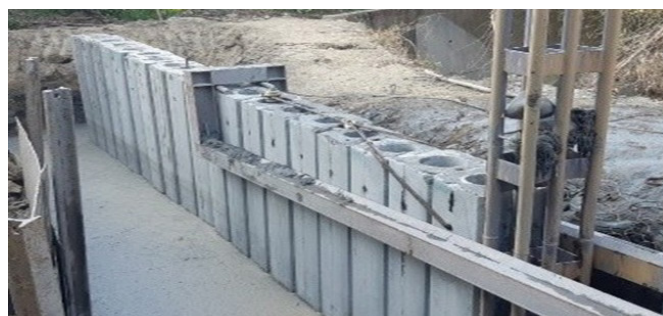
Fig. 2-1 Pile driving applying vibrators
