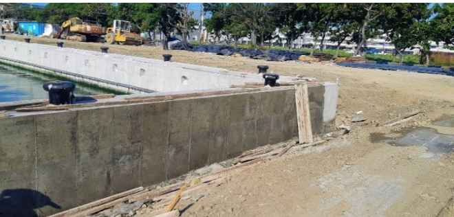
Fig. 2-4 Coastline retaining wall
