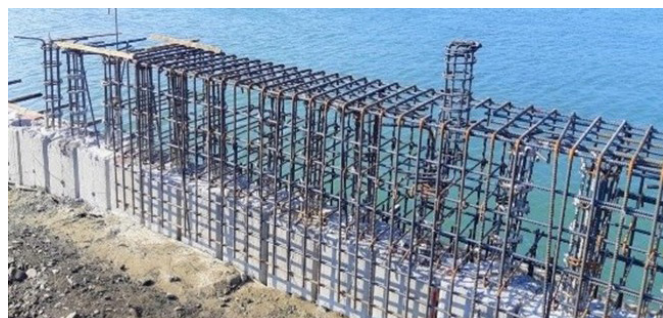
Fig. 2-2 Pile heads rebar works
