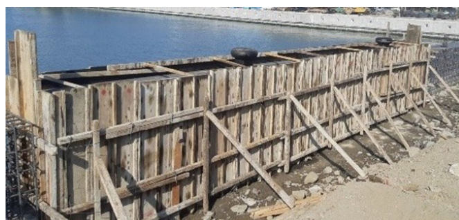
Fig. 2-3 Pile heads form works
