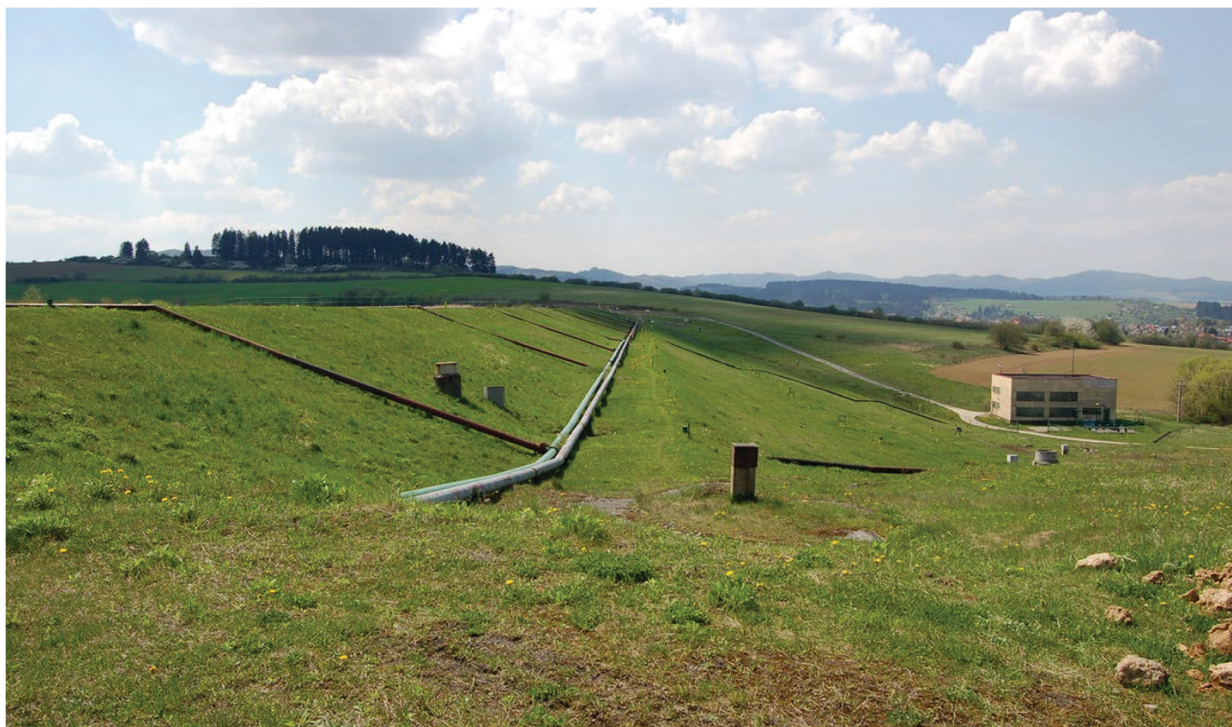
Fig. 4 The side view of the dam system of the Rosina tailings pond
