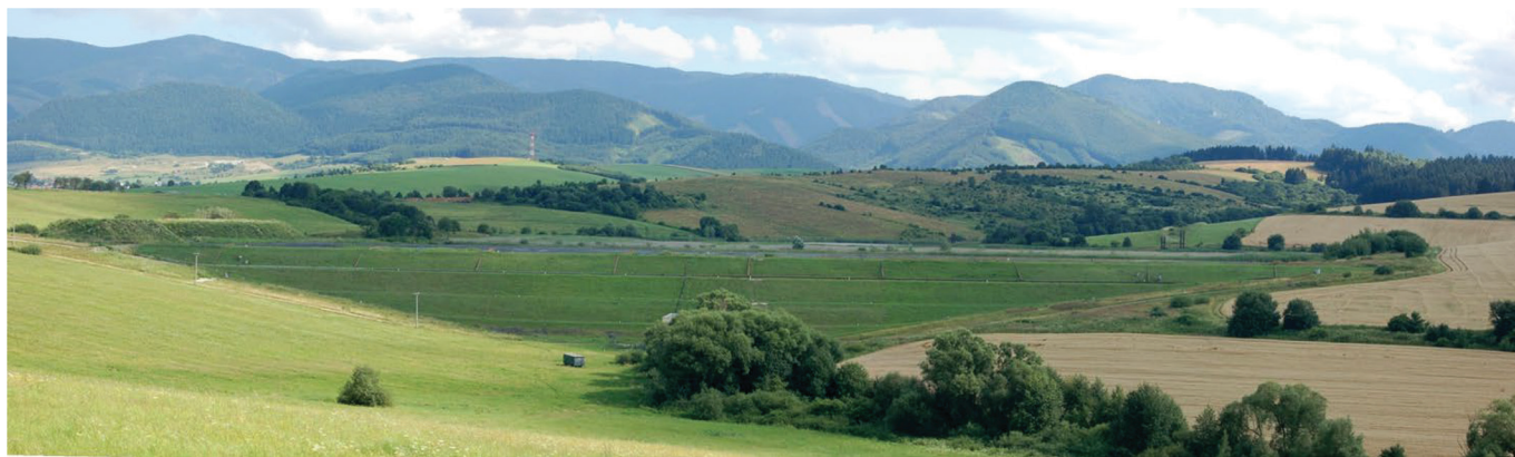
Fig. 3 Front view of the dam system of the Rosina tailings pond
