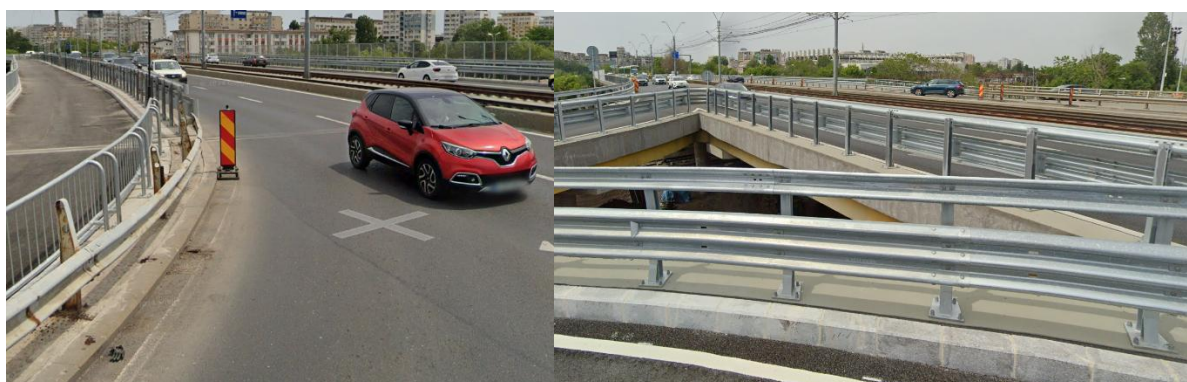
Figure 2. Grant Bridge Shoulder view when entering the traffic flow
