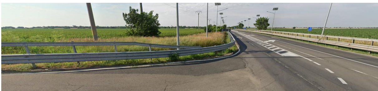
Figure 1. Low impact level guardrail in the intersection between National Road DN2 and county road DJ 203C
