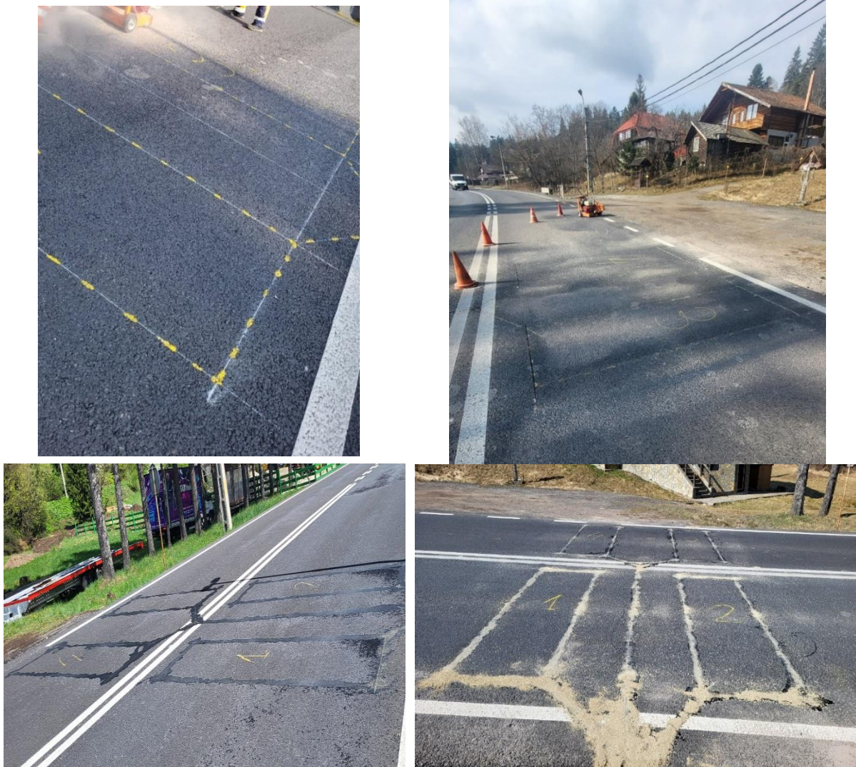
Figure 9. Installation of inductive loops in the roadway VEKPI - count
