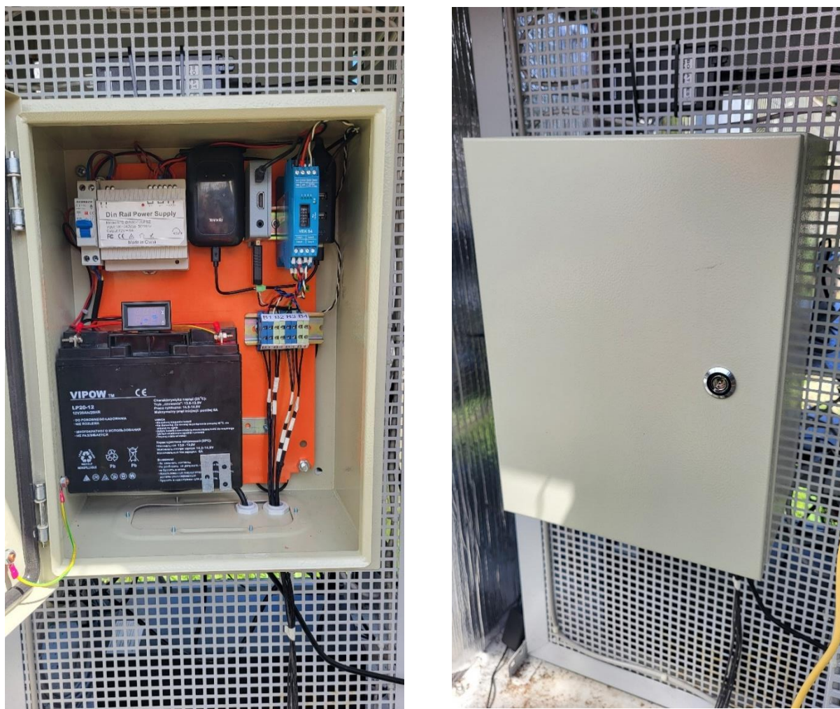
Figure 10. Installation of VEKPI– count - traffic counting equipment
