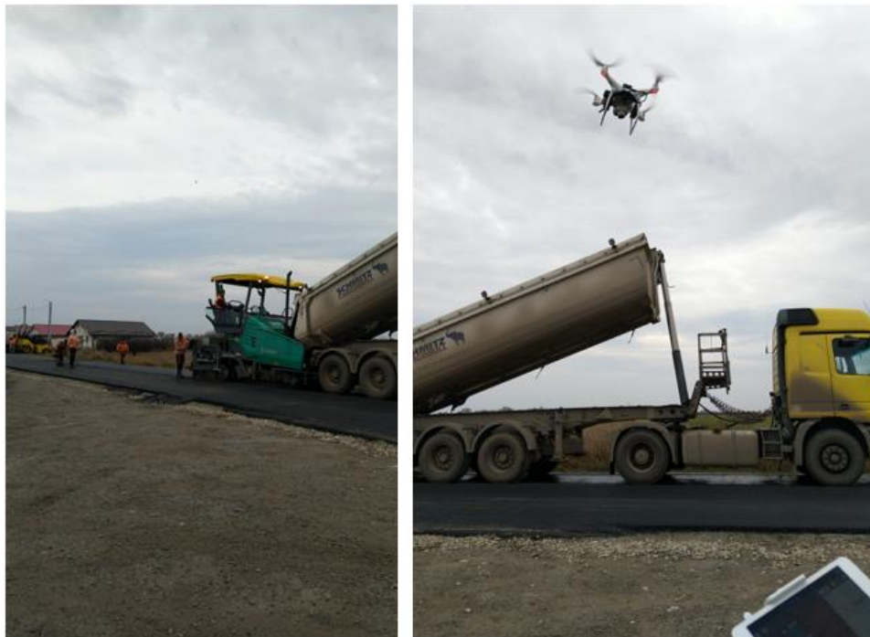
Figure 3. Bituminous layer laying
