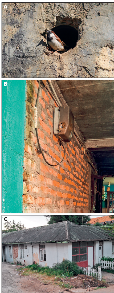
Figure 6. Different nesting substrates used by House Sparrows (A) Holes on walls (B) Light meter box (C) Gutters (see the edges of the roof)
