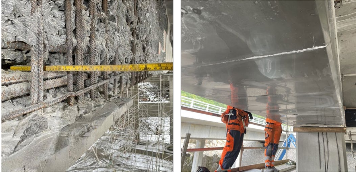
Figure 5 – Beam on Bukkestein Bridge before (left) and after (right) repair with UHPFRC.
