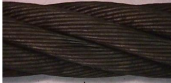
Fig. 4 An example of corrosion on a rope
