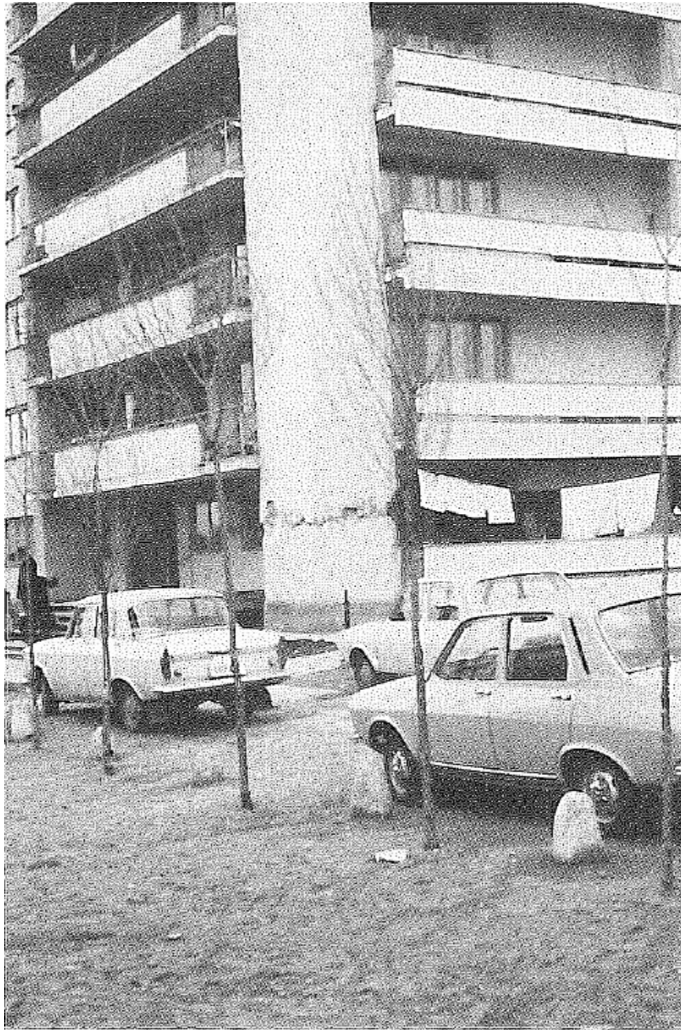
Fig. 3.8 - GF+10E Building Damaged in the Valea Roşie District [8]
