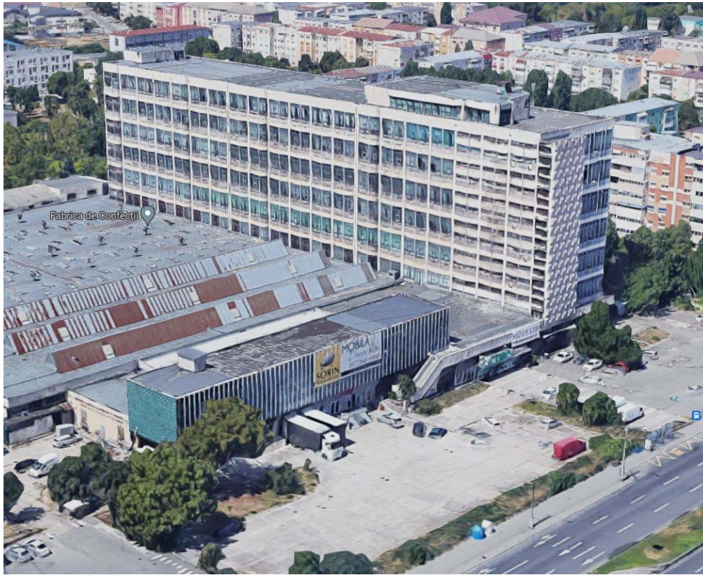
Fig. 3.16 - The Garment Factory Building
