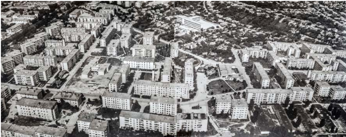
Fig.3.6 - Buildings in the Valea Roşie district – 1975
