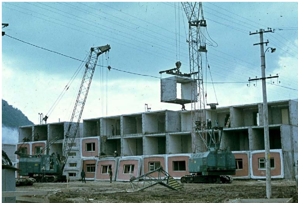
Fig. 3.15 - “Spatial Boxes” produced at the Prefabricated Components Factory in Braşov
