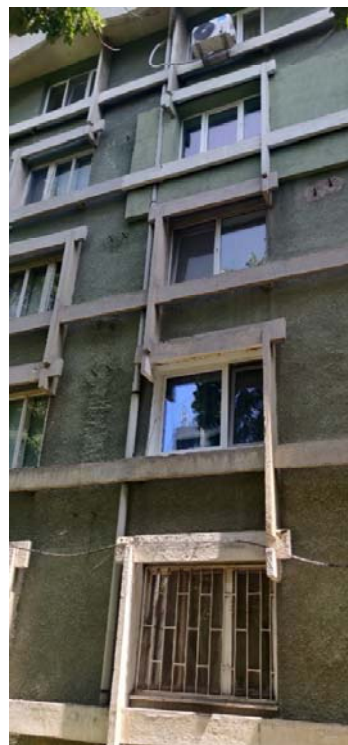
Fig. 3.10 - Tie rods on the exterior wall of Block A
