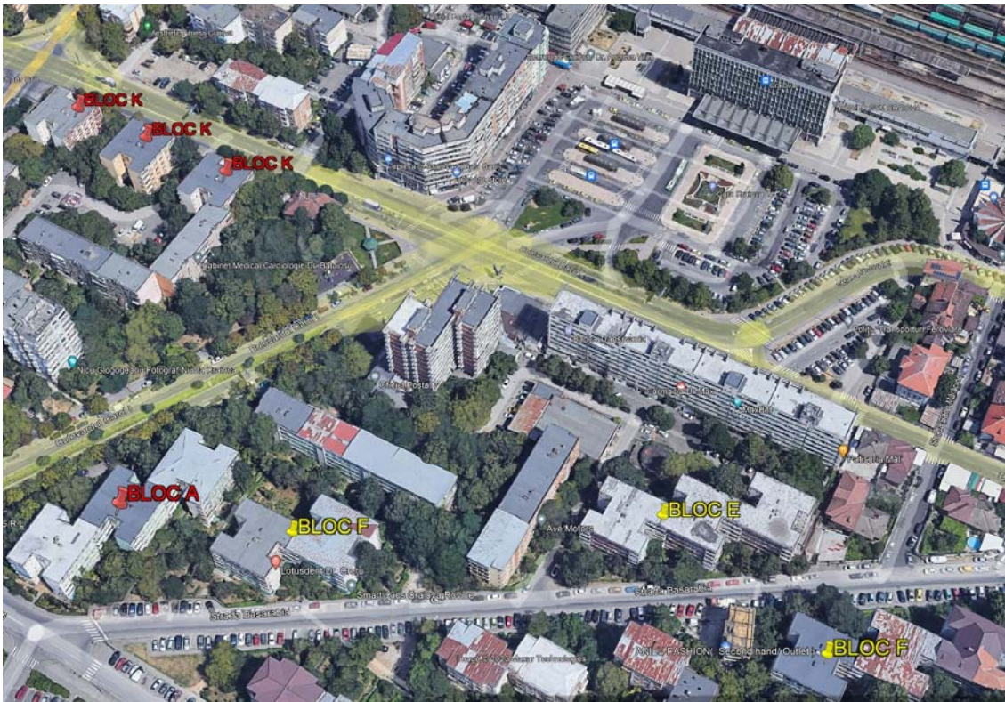
Fig. 3.9 - Typology of Damaged Buildings in the Piața Gării District
