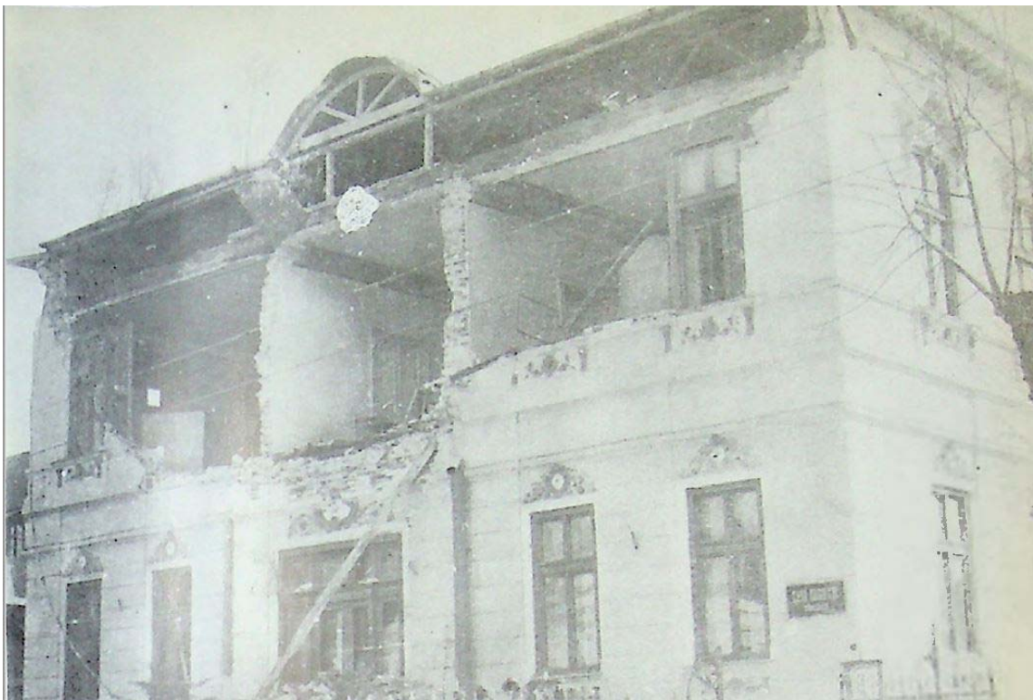
Fig. 3.11 - Damaged buildings in the central area of Craiova [5]
