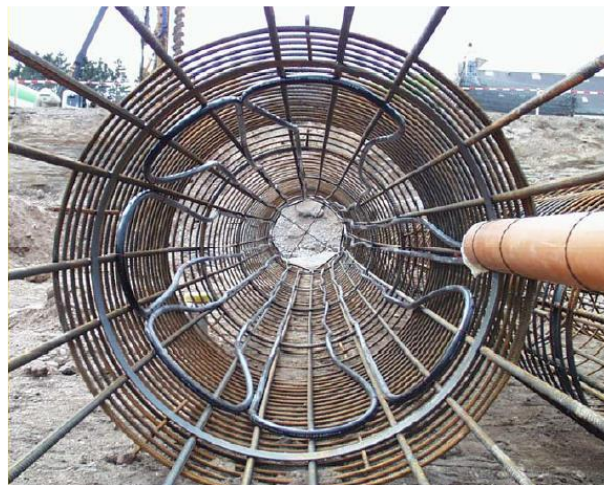
Fig. 4 - Reinforcement cage of an energy pile equipped with HDPE pipes
