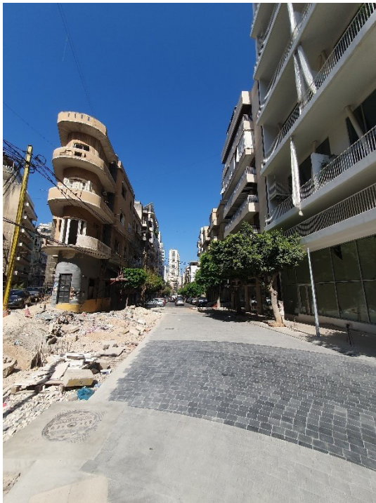
Figure 6. Halted construction works on The Mar Mikhael Square, 1 August 2023 Source: photo by author
