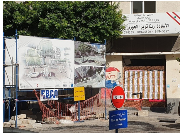
Figure 7. Banner with visualizations of the project on the construction site, 1 August 2023 Source: photo by author
