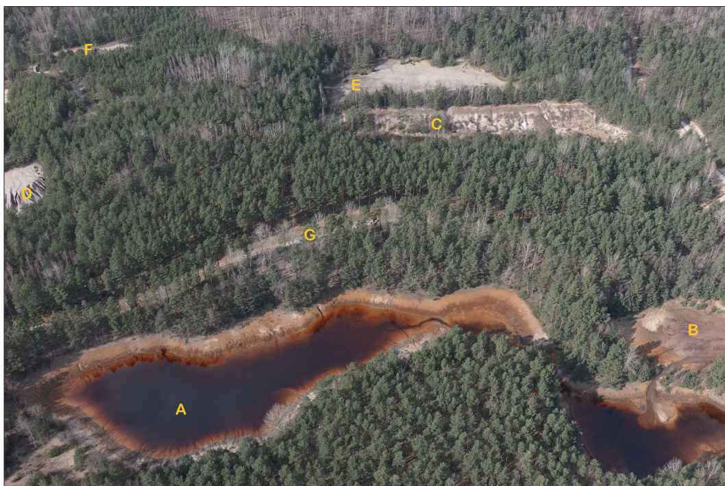
Fig. 12: Contemporary view of the southern part of the study area taken with drone photography. The letters indicate: A. flooded former brown coal open-pit, B. part of the former brown coal open pit filled with waste material from another excavation, C. former brown coal open-pit, partially filled with water, D. external, exposed, waste heap, E. external, exposed, waste heap, F. zone of former underground mining, G. present-day road (tourist educational trail). Photo: M. Becker (2024)
