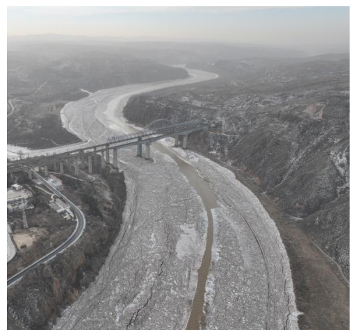
Fig. 1. Photograph of tandem double piers under ice-jammed conditions.
