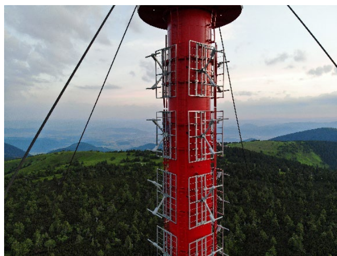
Fig. 1. Placement of a large antenna system on a monopipe structure
