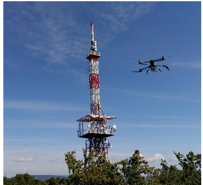
Fig. 8. Pixla 1 mounted on a UAV – before the aerial measurement (illustrating in-situ measurement environment)
