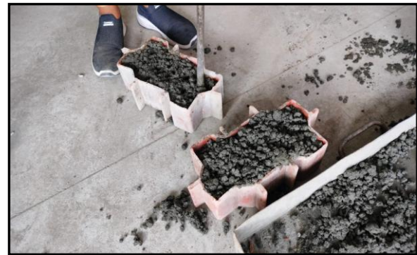
Figure 8. Casting of Paver Blocks
