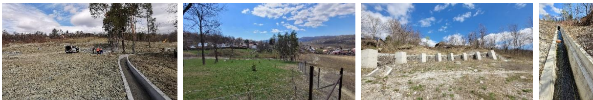
Figure 13. Site images after stabilization works
