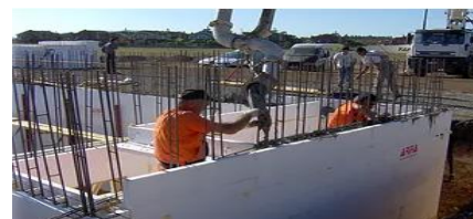
Figure 2. Construction Process of ICF Wall System (ARFA Construction Website)
