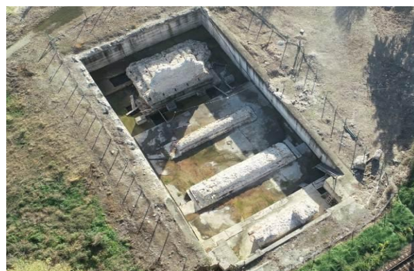
Figure 13. Water infiltrations present in the monument area
