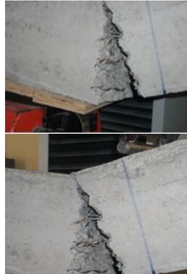
Figure 15. Example of failure mode of series 2 beams
