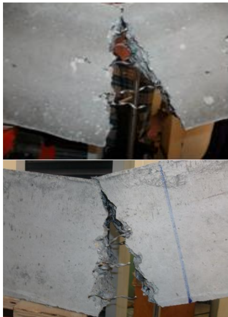
Figure 17. Example of failure mode of series 3 beams
