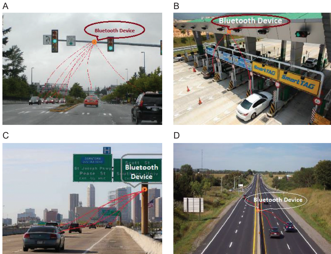
Figure 4: (A) Bluetooth device, installed at the traffic light, (B) Bluetooth device, installed at the toll booth entrance, (C) Bluetooth device, installed at the banner stand, and (D) Bluetooth device, installed at the road divider.
