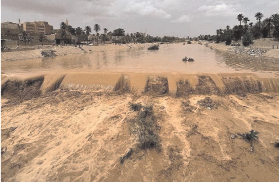
Fig. 1. Flood event on September 10, 2024, in Oued Bacher, located in the southwest of Algeria (photo by Melina Malek)
