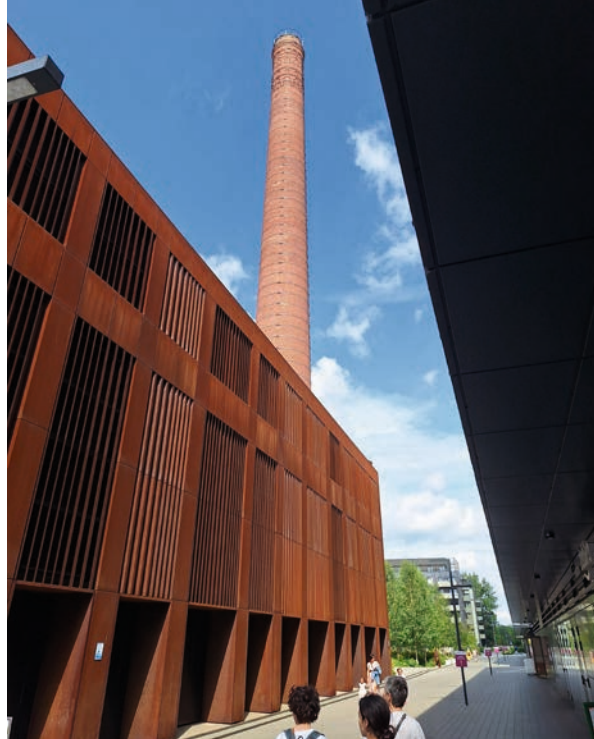
III.9. Łódź, new Corten steel facade of the former power plant, photo: M. Gyurkovich, 2025
