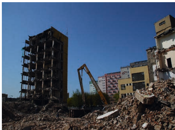
III. 6. Demolition of the buildings of the DANA Clothing Factory in Szczecin. Photo Z. W. Paszkowski
