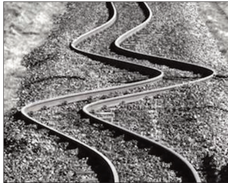
Figure 2. Railroad tracks bent due to linear thermal expansion (image source: https://thermtest.com/what-is-coefficient-of-thermal-expansion-how-to-measure-it ).
