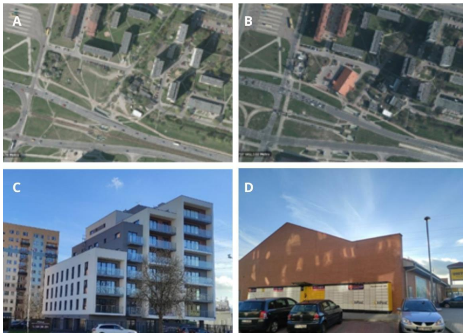
Fig. 5. Example of field verification of change detection in the Widzew Wschód housing estate in Łódź – (a) orthophotomap from 2017, (b) orthophotomap from 2021, (c) (d) photographs from 2023.
