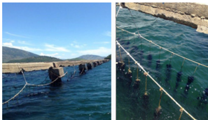
Figure 1. A "panel" type system, with concrete structures, for the cultivation of mussel ( M. galloprovincialis ) in Butrint Lake
