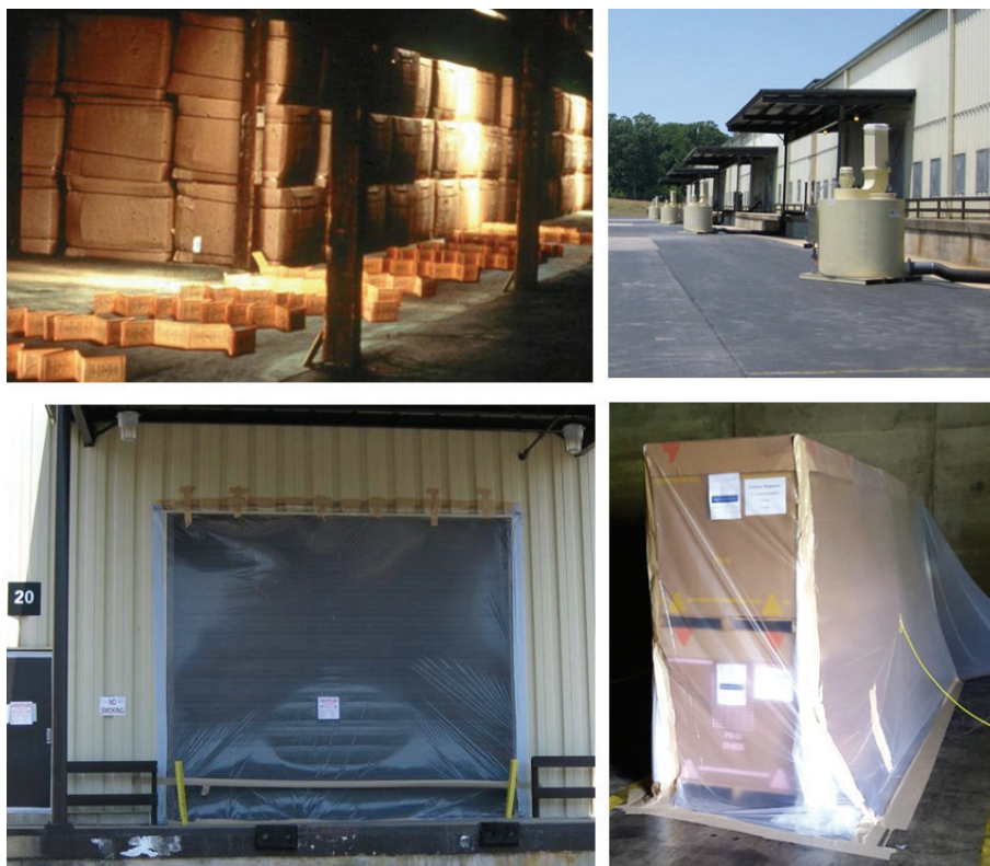
Figure 4. Gas-tight sealing for fumigation of stored tobacco showing typical situations for application of phosphine. Top-left is the inside of a warehouse prior to sealing openings to the outside, Top-right is a series of warehouses onto which windows have been sealed with thick cellophane and duct tape. Bottom-left is an example of a loading dock door that is sealed for fumigation. Bottom-right is a collection of a few boxes covered and sealed for localized, small fumigation.
