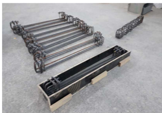
Figure 2: Reinforcement cages and beams formwork
