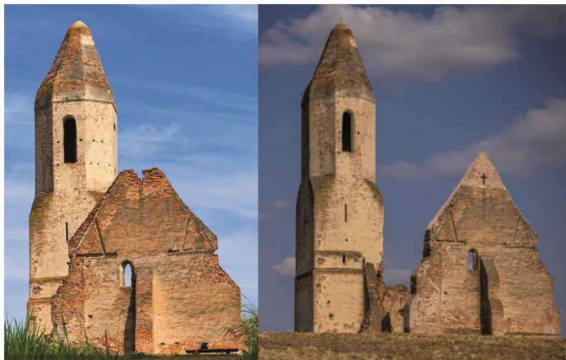
Figure 14: Pusztatemplom/Somogyvámos (Hu). The modification of the western wall clearly interprets the original architectural shape. The cross sign in the negative of the masonry is added. Before and after restoration. Sources. Left: Joó, 2024. Right: Farkas, 2024
