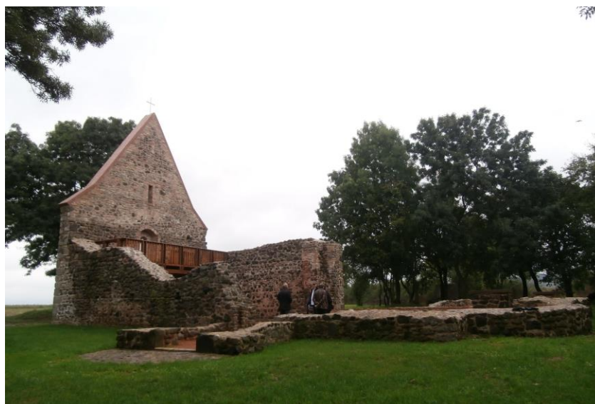
Figure 22: Realized renovation of the church from south, 2014. Photo: B. Polomová
