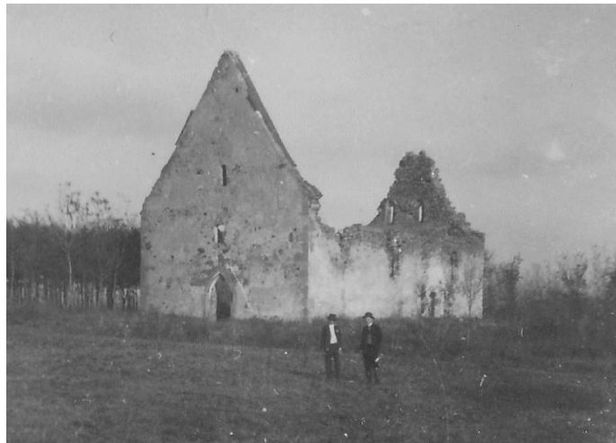
Figure 10: Church in the year 1935. Source: Archive of the municipality Velká Čalomija
