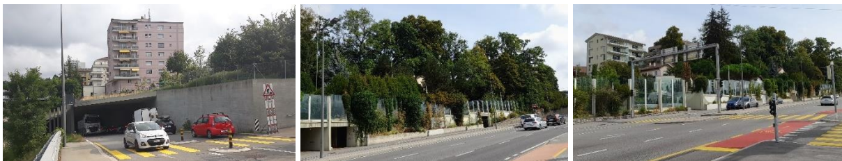
Figure 14: Photographs from year 2022 of Road traffic noise reducing devices combined with green infrastructure, Lausanne (Píry et al., 2023)
