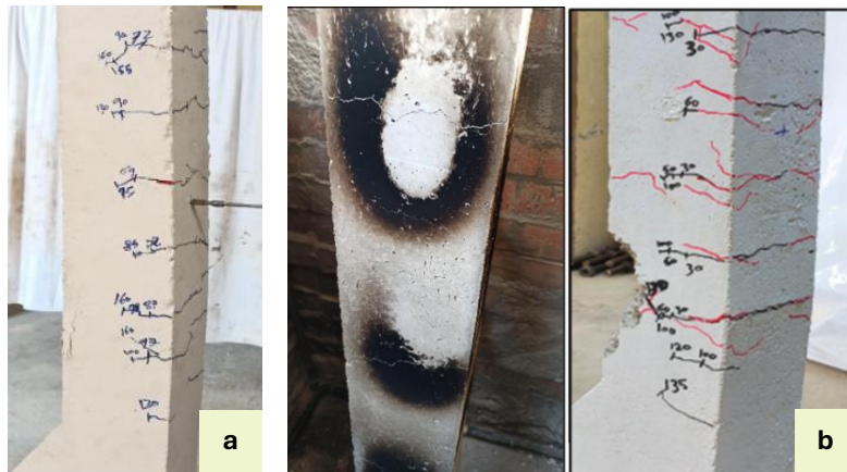
Figure 15: Spread of crack in specimens, a. Column specimens without fire, b. Column specimens with fire exposure
