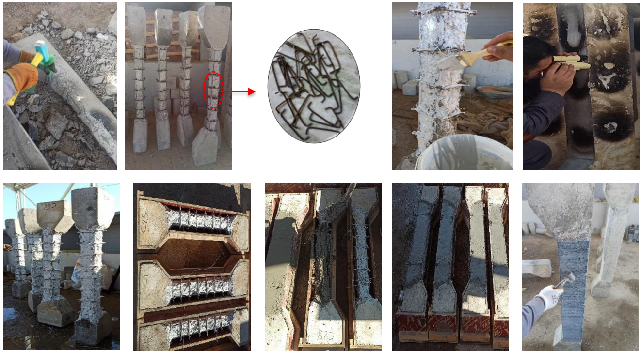
Figure 6: Sequential steps of RC column repair
