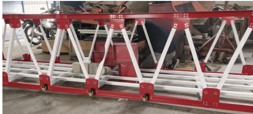
Figure 10: Experimental simulation of mid-span diagonal member damage (Dmg-CC)
