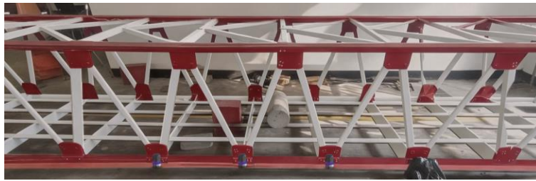
Figure 19: Experimental simulation of diagonal member damage at 1/5 of the span (Dmg-CE)
