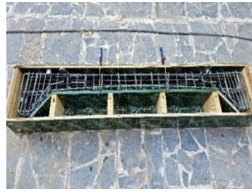
(b) Reinforcement gage in mould
