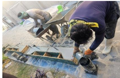
(e) Moulds filled with concrete
