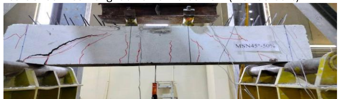
f) Failure mode of a 50% pre-damaged beam strengthened by CFRP bars at 45° near longitudinal reinforcement (MSN45-50%)
