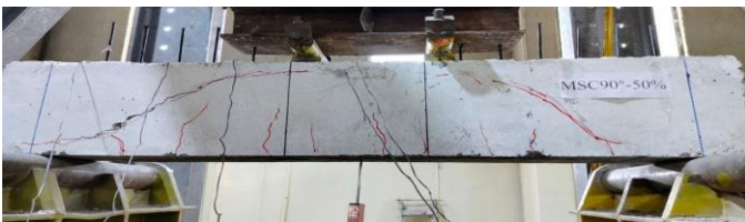
g) Failure mode of a 50% pre-damaged beam strengthened by CFRP bars at 90° in the center (MSC90-50%)
