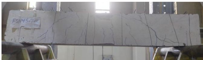
e) Failure mode of a 70% pre-damaged beam strengthened by CFRP bars at 45° near longitudinal reinforcement (FSN45-70%)
