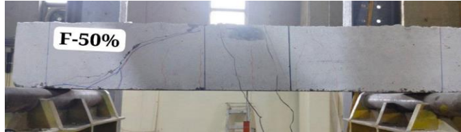
a) Failure mode of a 50% pre-damaged beam (F-50%)
