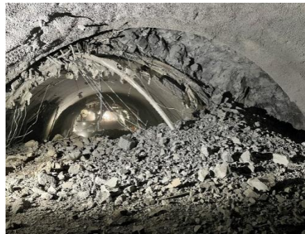
Figure 3: Revealed rock mass during expansion of Tingxin tunnel
