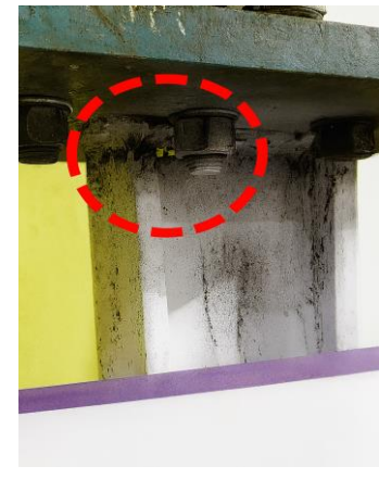
Figure 13(i), Failure condition: fracture at the upper weld region (specimen LL-2, 9B Cycle).
