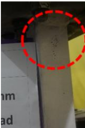
Figure 13(d), Yield condition: paint flaking observed on the flange section (specimen LL-1, 6B Cycle).
