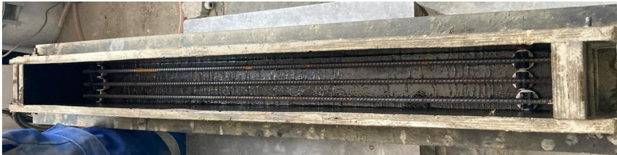
Figure 9: Mold with inserted reinforcement prepared for beam casting
