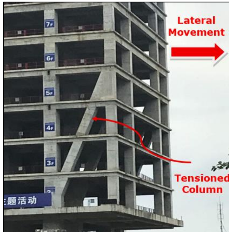
Figure 1: Reinforced Concrete Tensioned Column
