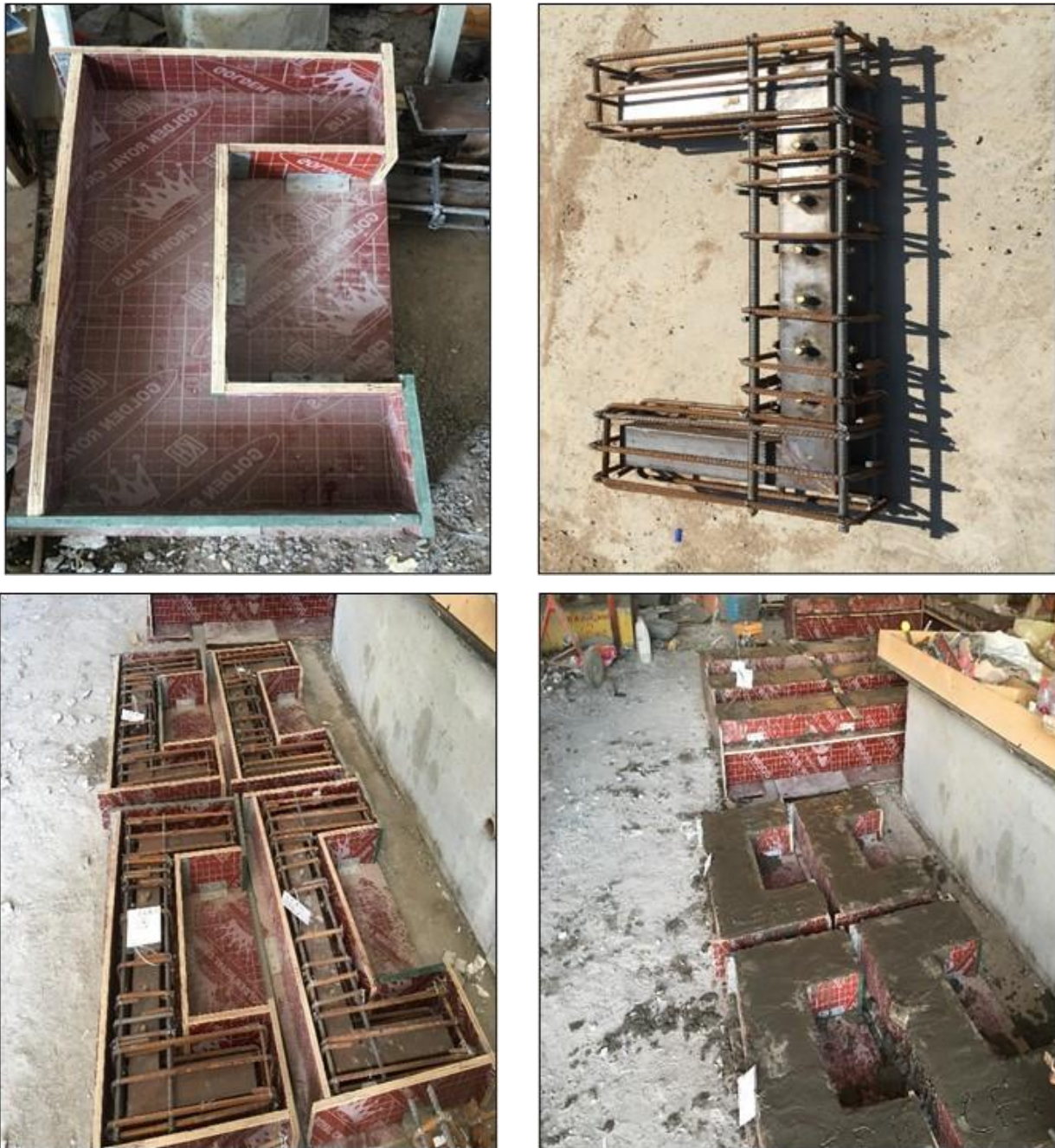
Figure 5: Fabrication the Specimens
