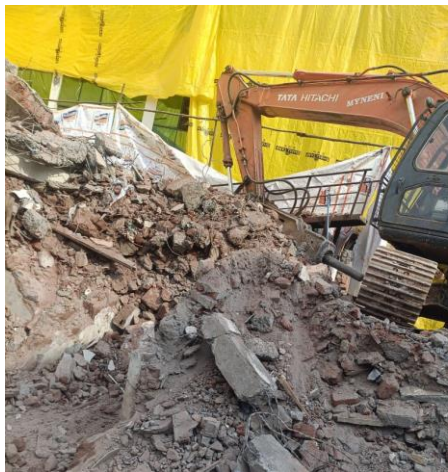
a) Construction demolition waste
