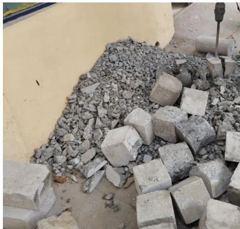
b) Sort waste concrete and artificial crush
