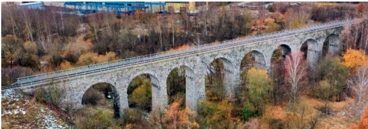
Figure 6: Viaduct Milevsko – view from a drone
