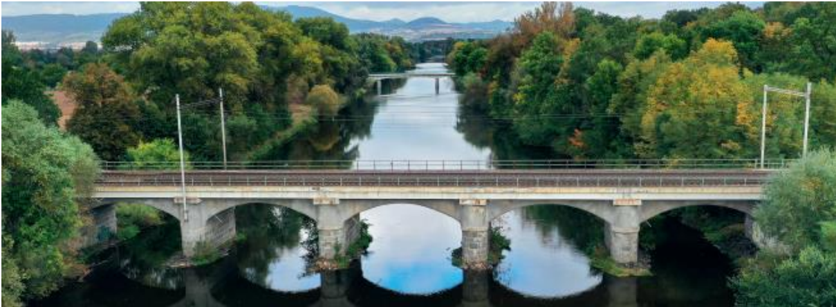
Figure 5: Bridge over the Ohře River in Bohušovice – view of the bridge
