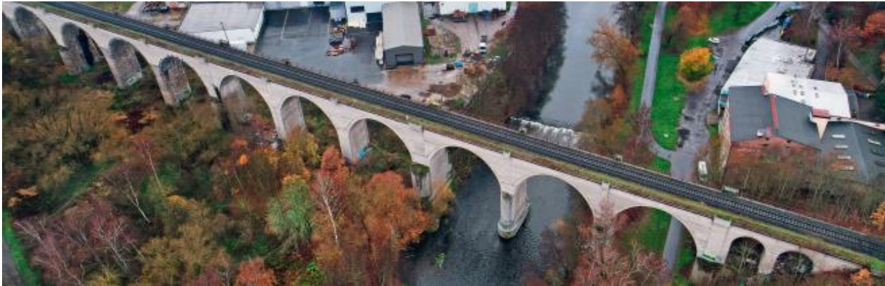
Figure 4: Cheb Viaduct – view from a drone
