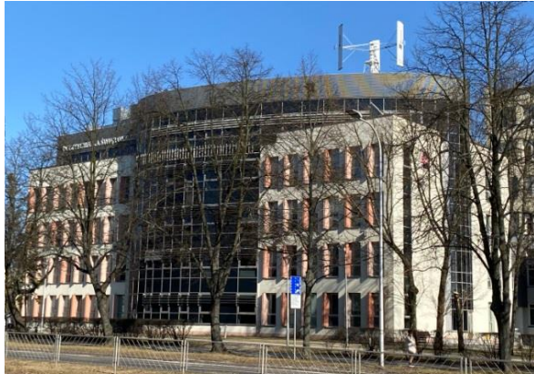
Fig. 1: Photo of the smart building „Energis”.
