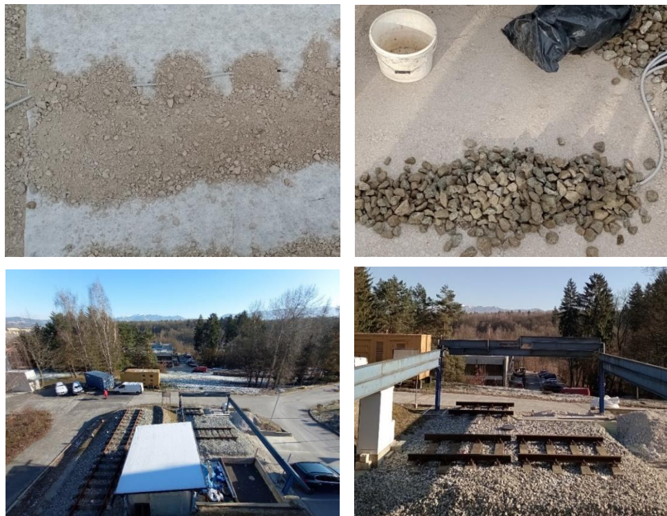
Fig. 6: Construction of MP8 – application of drainage geocomposite on the subgrade surface level with installation of temperature sensors (top left), installation of temperature sensor at the level of the sub-ballast upper surface (top right), overall view of the DRETM Test Stand (bottom left), detailed view of MP8 (bottom right).
