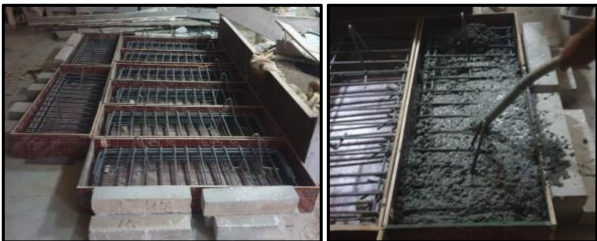
Fig. 4: Steel Reinforcement of deep beams.
