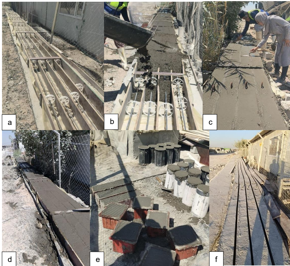
Fig. 1: a) The formwork, b) during casting, c) leveling the surface, d) and e) after casting, d) the hardened 30m beams.
