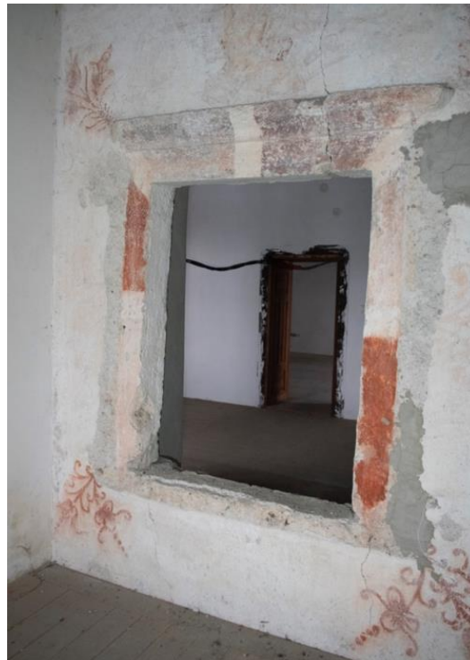
Fig. 5: Early Renaissance window from the first construction phase of Trebostovo manor house. Author: Krušínský.
