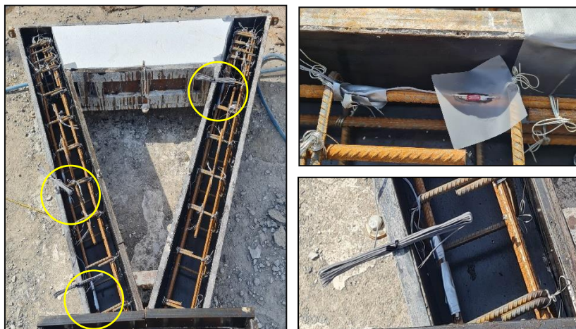
Fig. 4: Strain gauges for steel reinforcement bar.
