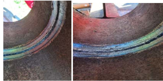
Figure 6. Examination of weld penetration
