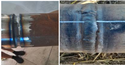
Figure 4. Checking the cleaning of slag between layers
