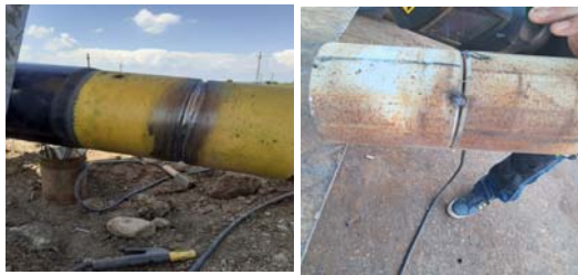
Figure 3. Visual testing of welded joints
