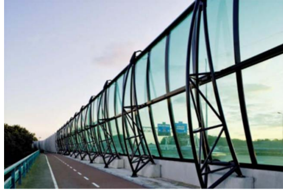
Fig. 4 – Phonoabsorbent panels made of plastic materials (Ștefan, 2018).
