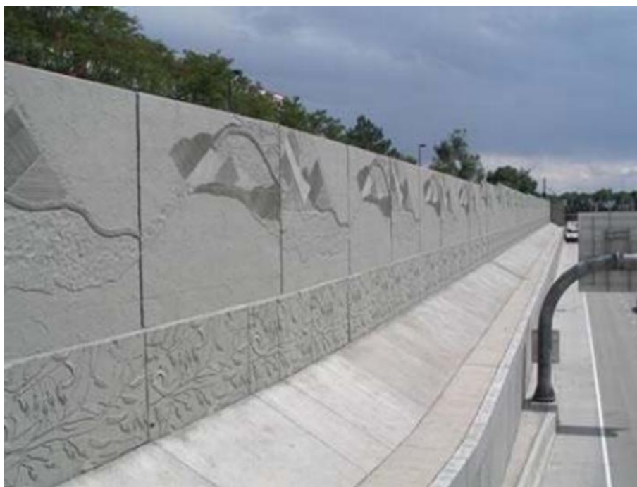
Fig. 3 – Reinforced concrete phonoabsorbent panels (Ștefan, 2018).
