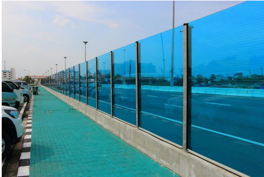
Fig. 2 – Acrylic glass phonoabsorbent panels (Ștefan, 2018).
