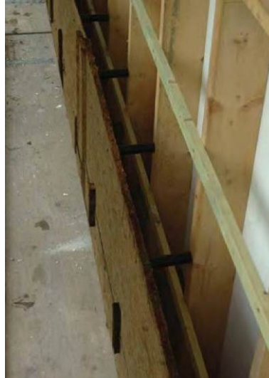
Fig. 5 – The internal exposed frame for permanent shuttering, featuring horizontal rails (Zuo, 2021).
