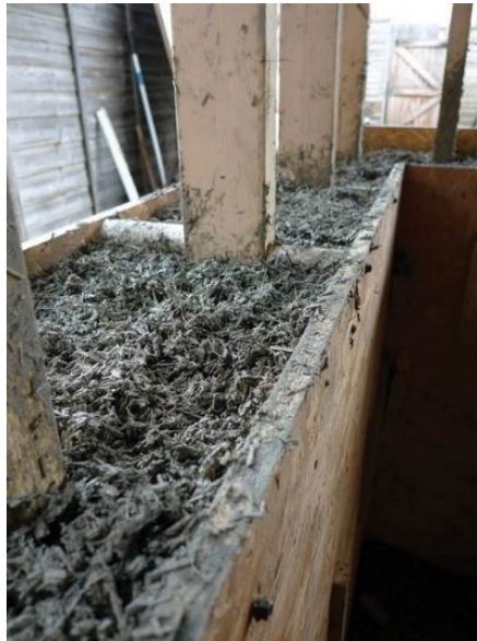
Fig. 4 – Softwood frame centrally embedded within the wall (Stanwix & Sparrow, 2016).
