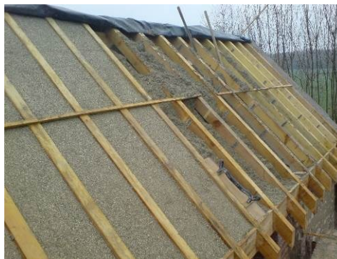
Fig. 8 – Hempcrete roofing (Tradical, 2017).
