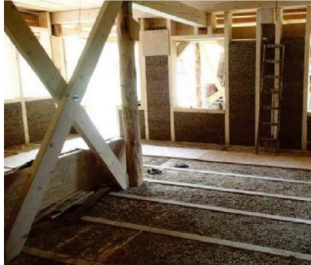
Fig. 7 – Hempcrete walls and flooring (Madhura & Ayushi, 2022).
