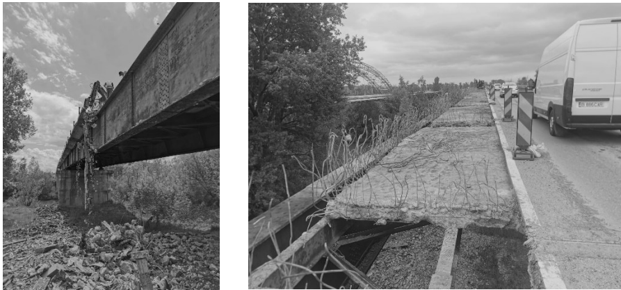
Fig. 5 – Demolition of reinforced concrete decking
