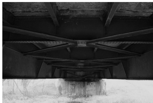
Fig. 2 – The metal bridge superstructure
