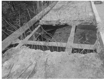
Fig. 3 – The “collaboration” between the metal structure and the reinforced concrete deck
