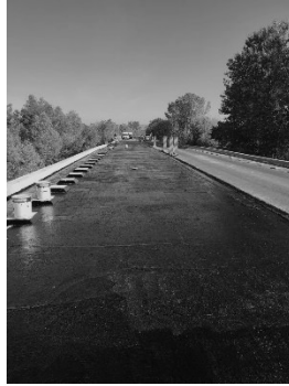
Fig. 7 – Priming the support layer
